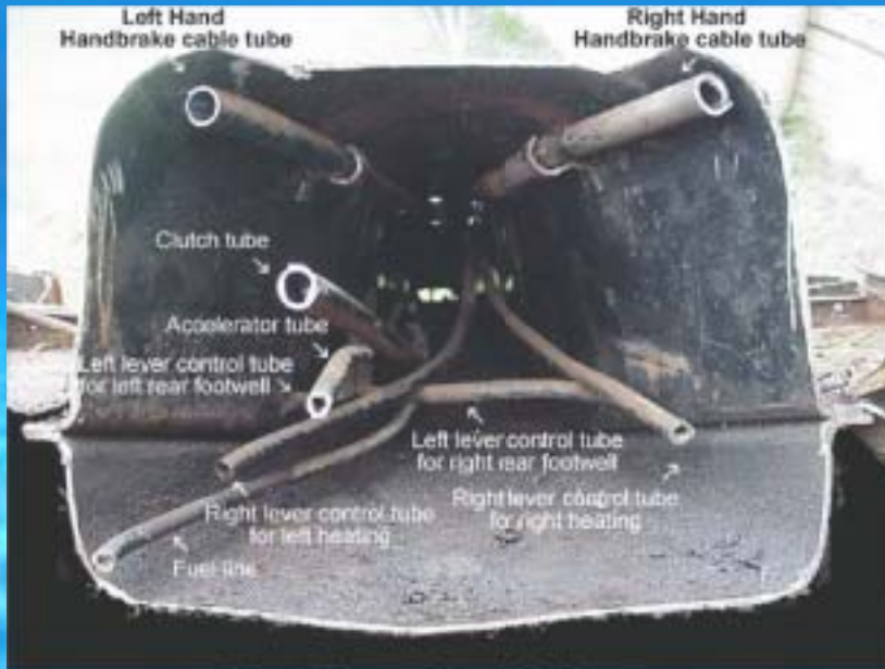
Peering into the tunnel from just in front of the rear torsion tube (which has been removed) top of page
