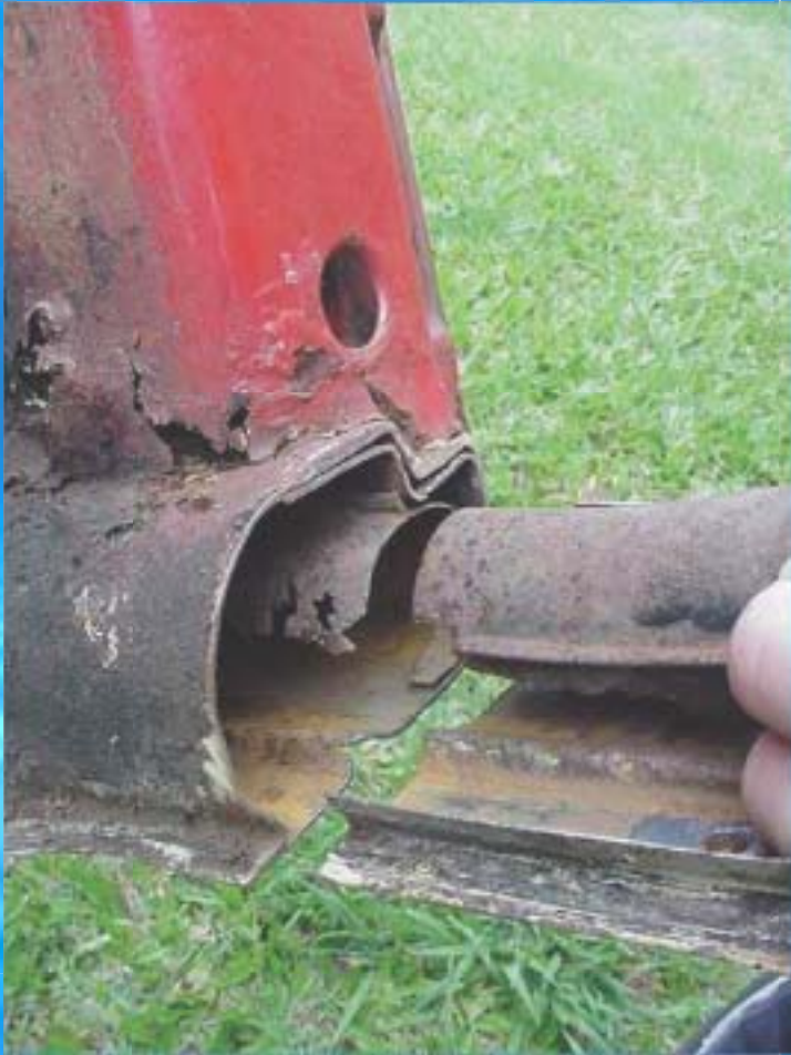
The right hand heater channel where it meets the "A" pillar. The heater duct at this point is socketed into each other (I did not cut the duct at this point). The top of the heater channel on the right of this photo has been removed to expose the heater duct inside. top of page
